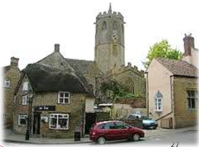
Figure 18: South Petherton village centre
